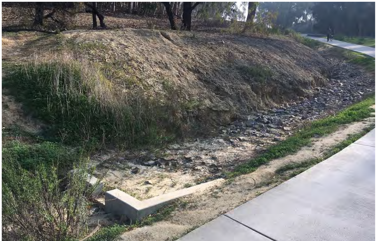
Close-up of damaged swale filled with mud and debris. Clogged drainage structure and example of erosion of adjacent slope.
