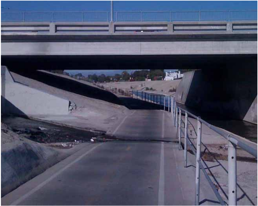
Ballona Creek Path : 12' wide - Concrete
