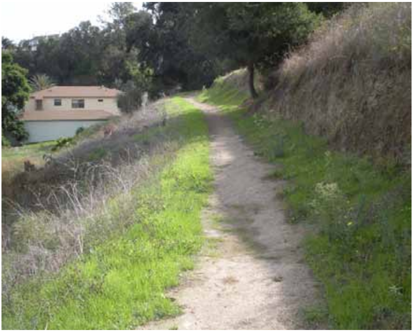
Stocker Corridor: 3'-5' wide - Compacted earth
