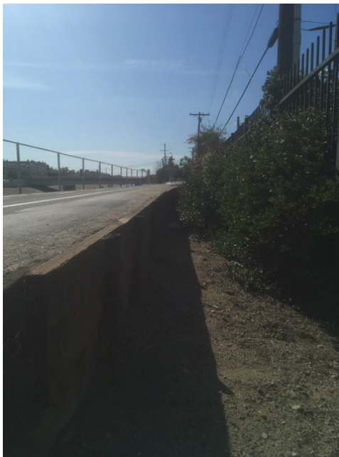
Pictured here is where DG path extensions were added to widen the path for the benefit of pedestrians, but created an unintended consequence of a tripping hazard.
